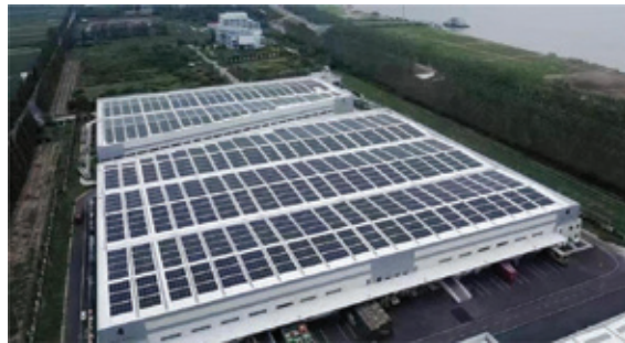
Hannan Jieyue hang Photovoltaic Power Generation Project
